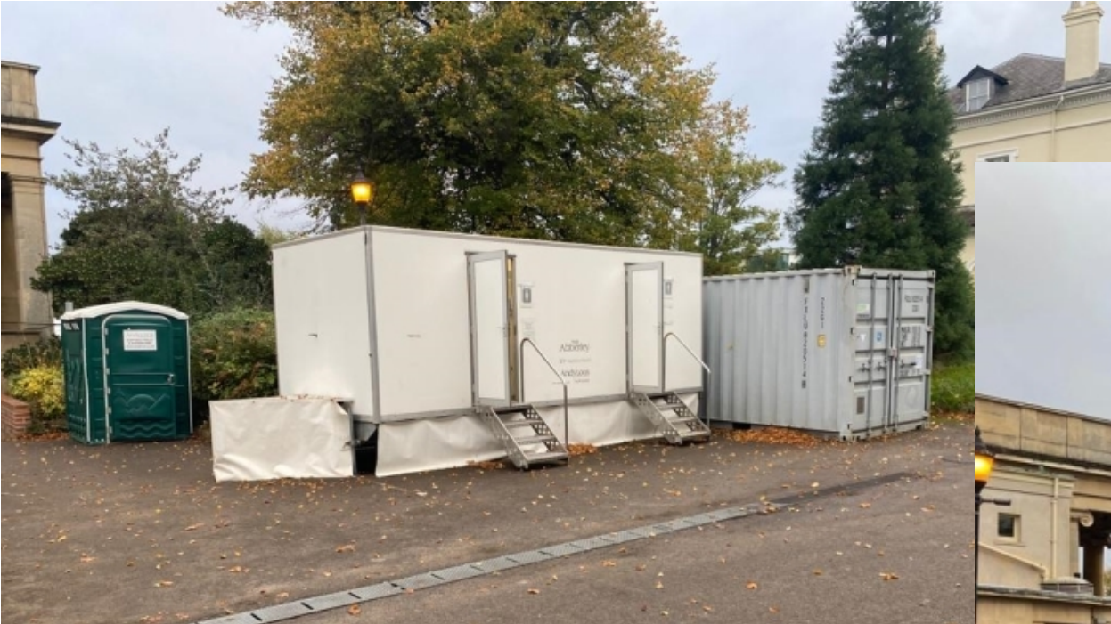
Site photos – Toilet block and storage container located within the rear of the building
