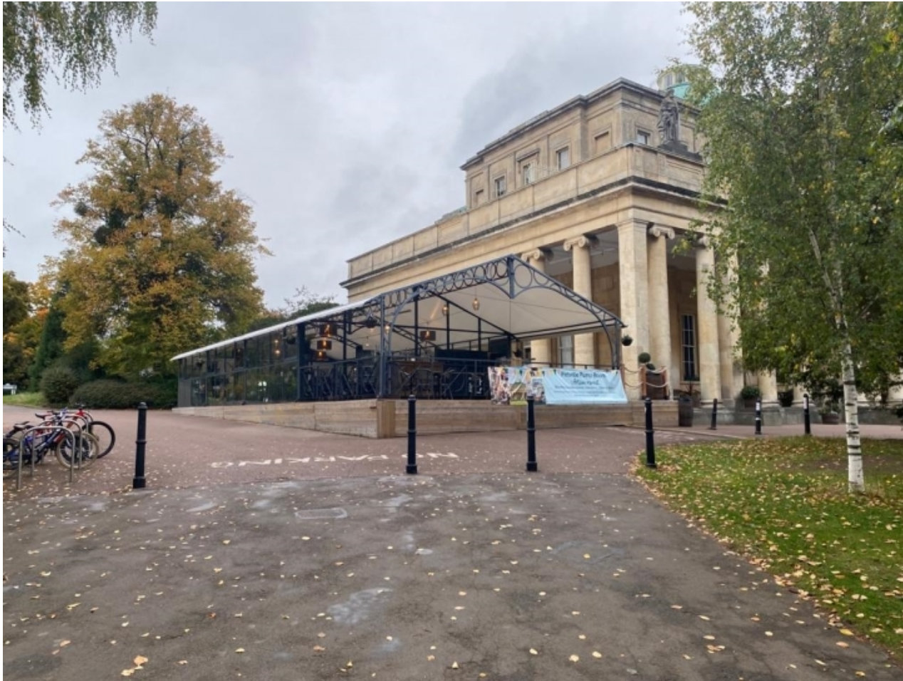
Site photos – Views of the Orangery from within the park
